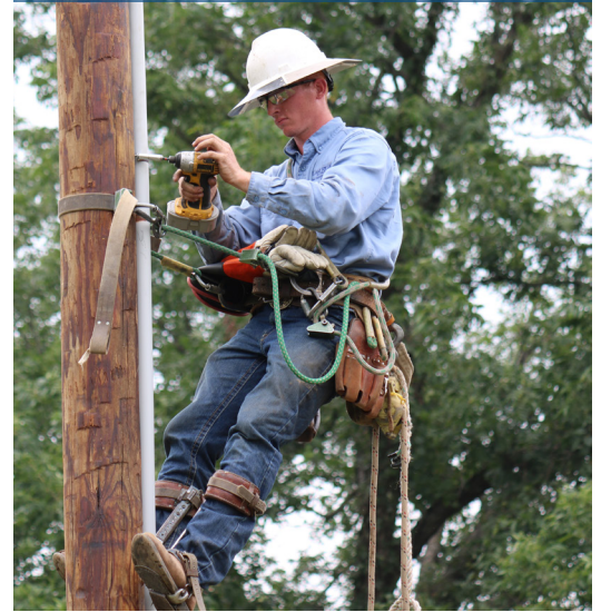
Kane Teague, Apprentice Lineman
